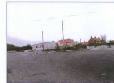
The Former Highway Depot
