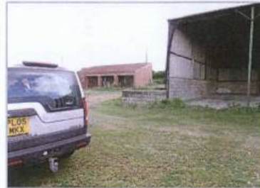
The Farm Buildings On Outgang Road
