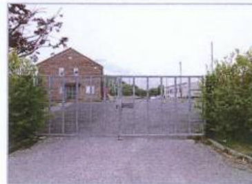
The Former Highway Depot
